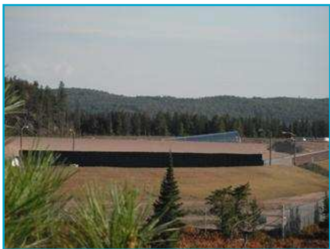
Portal construction at Eagle Rock, September 2011.
