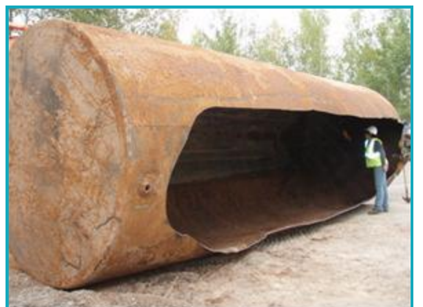
Tank #1 removed and being cleaned.
