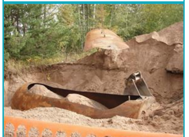
Tank #2 in the ground filled with sand.
